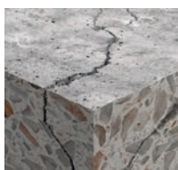
Cracked concrete
